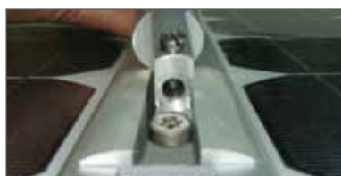
Apply the tool with the milling groove on the screw.
